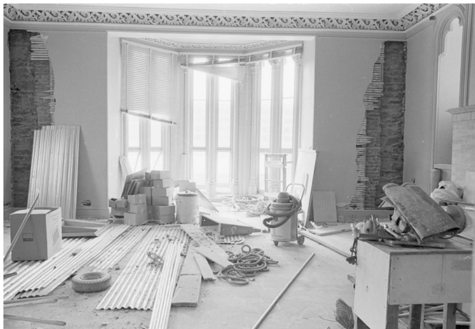
Figure 6: Photo of Regent's Room renovation circa 1968 showing exposed interior wall construction.
