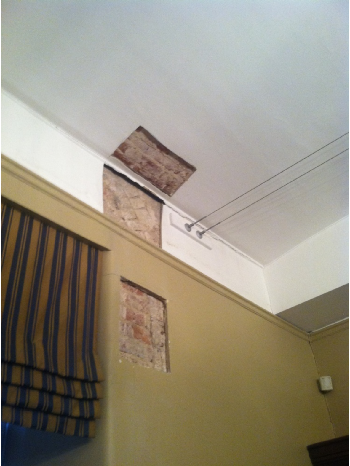
Figure 3: Probe west of window in Secretary's Office ("above the printer" location).
